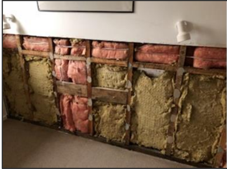
Figure 4: Gyprock partially removed to allow for investigation and formulation of design
