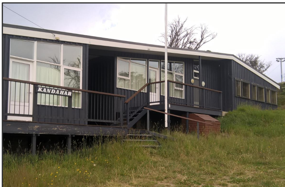
Figure1: Kandahar Ski Club (Source: Department inspection)
